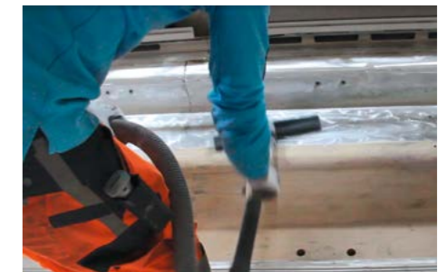
Traveller Installation SNCF Trains
